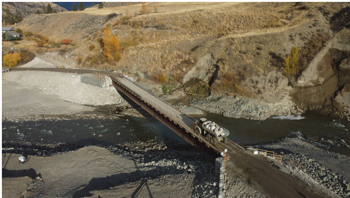
FIGURE 13: REPAIRS TO SITE 10D (Photo taken November 1, 2022)
