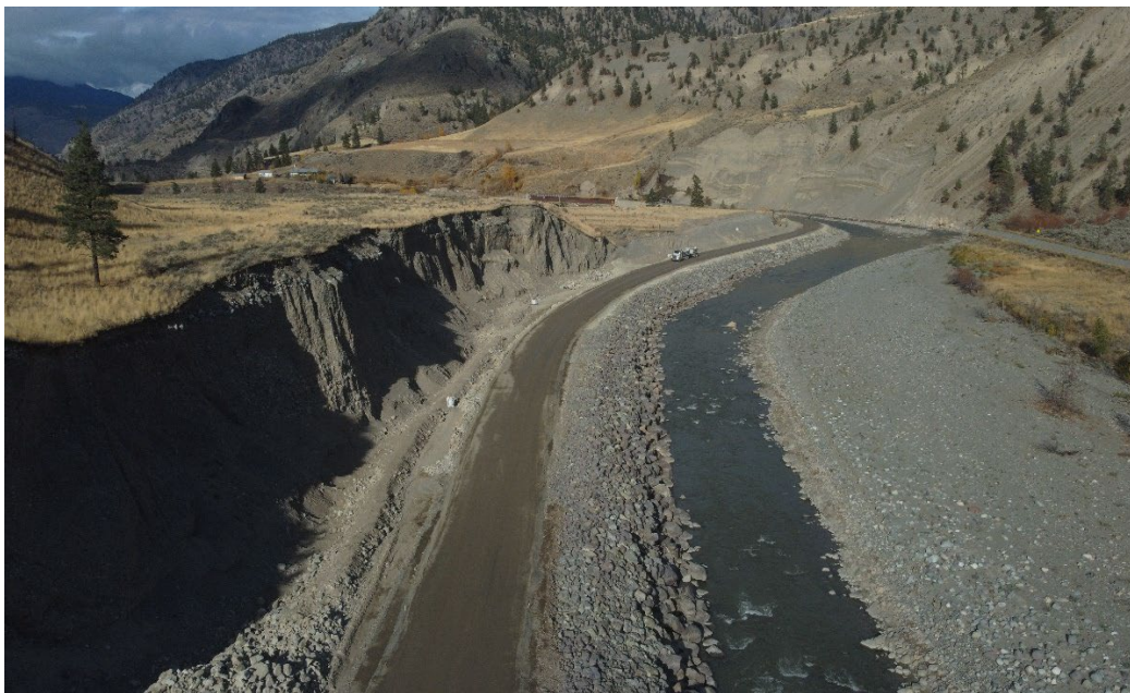
FIGURE 11: REPAIRS TO SITE 10C (Photo taken November 1, 2022)
