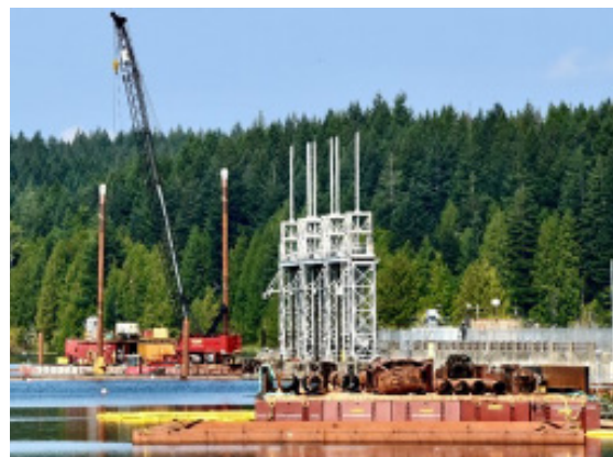
▶ John Hart Seismic Upgrade – Silt Installation
