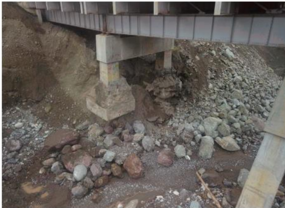
Figure 1 – Damage to Nicomen Bridge (Photo taken on November 24, 2021)
