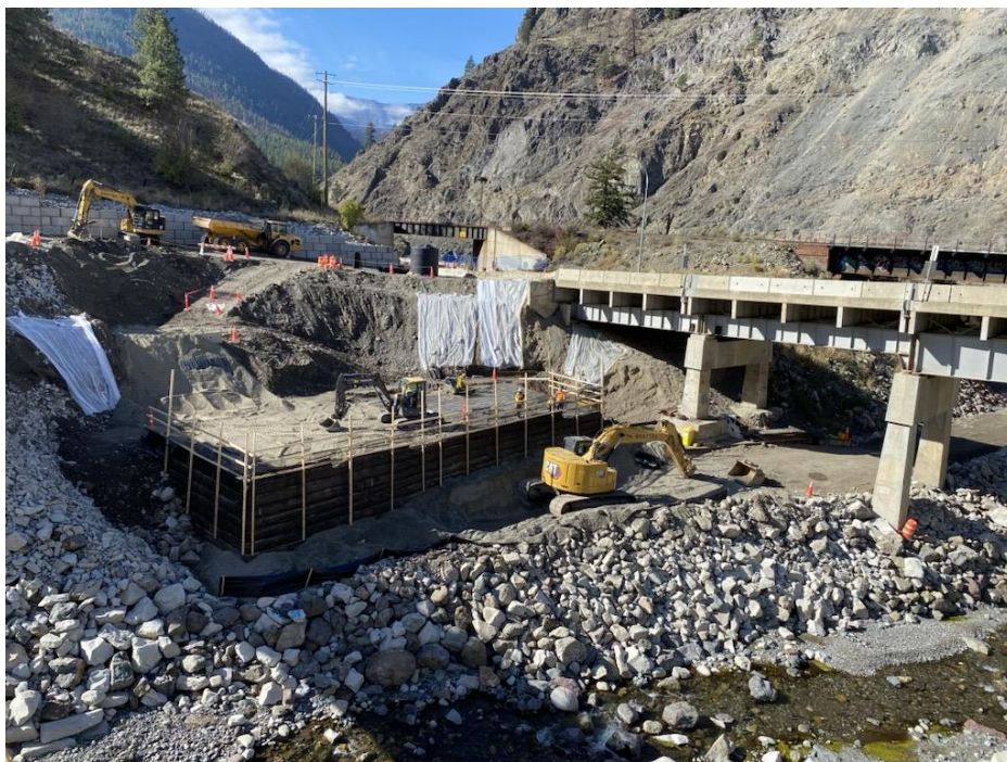
Figure 3 – Early Works Construction on South Embankment MSE Wall for Detour Bridge (Photo taken October 3, 2023)
