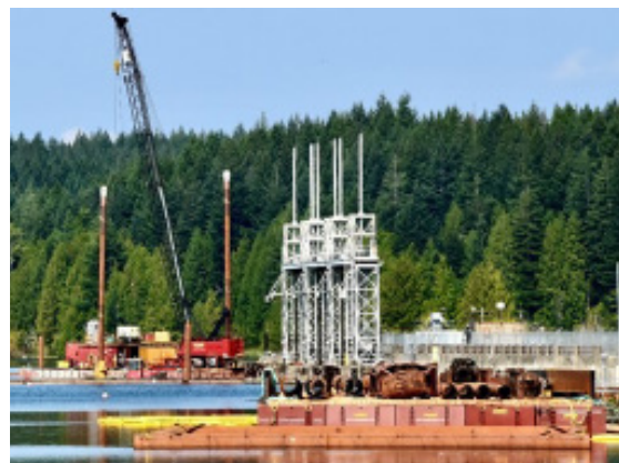
▶ John Hart Seismic Upgrade – Silt Curtain Installation
