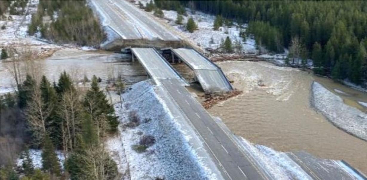
**Figure 6: Damage to Bottle Top Bridge (Photo taken on November 16, 2021)**
