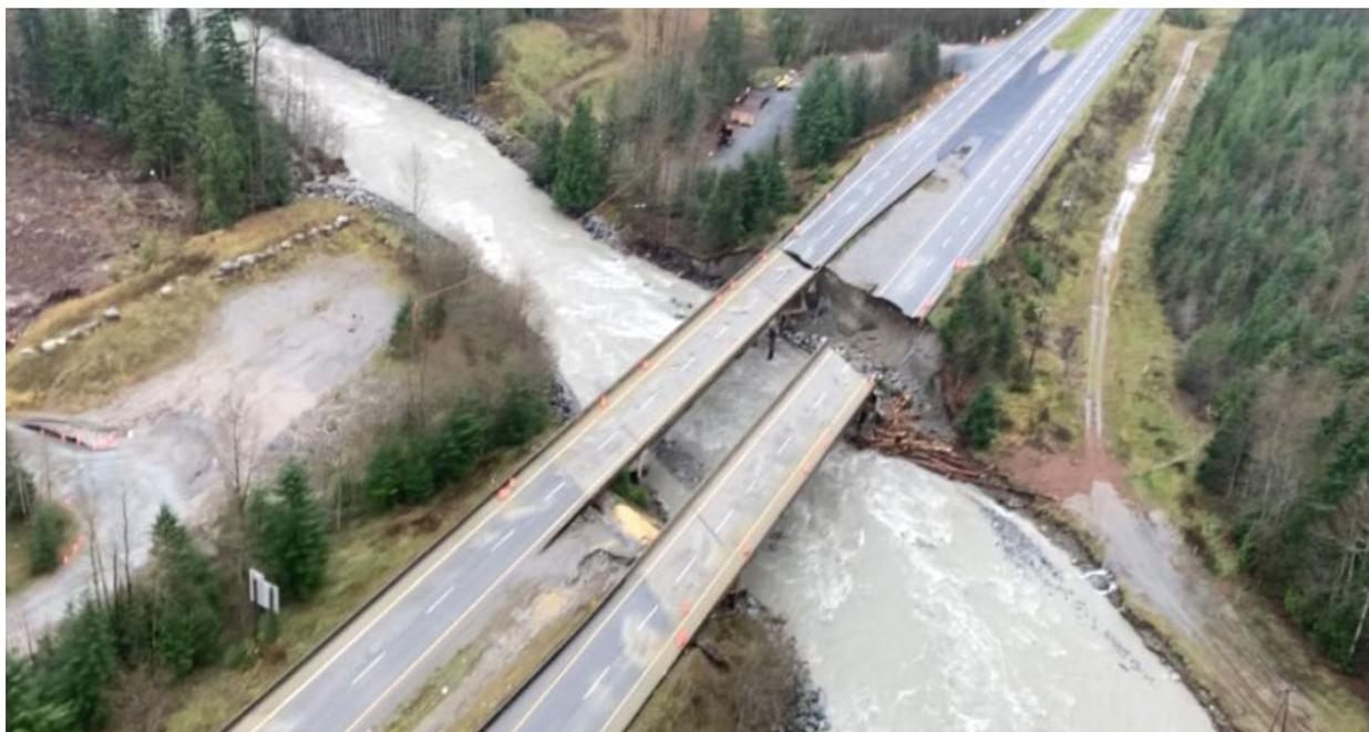
**Figure 3: Repairs to Jessica Bridge (Photo taken on December 14, 2021)**
