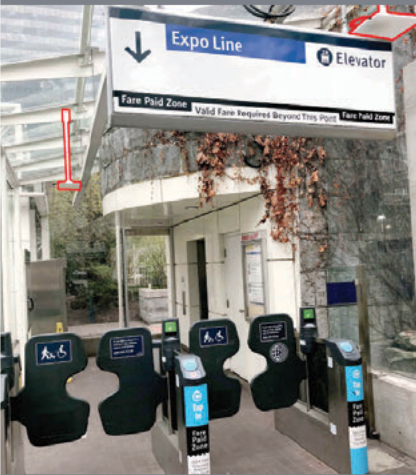
Fig 7.6 Example of Uni-Directional RFID Assemblies - RFID antennas can be seen installed and offset from each faregate (outlined in red).
