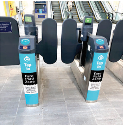
Fig 7.1 Example of a Standard Faregate
