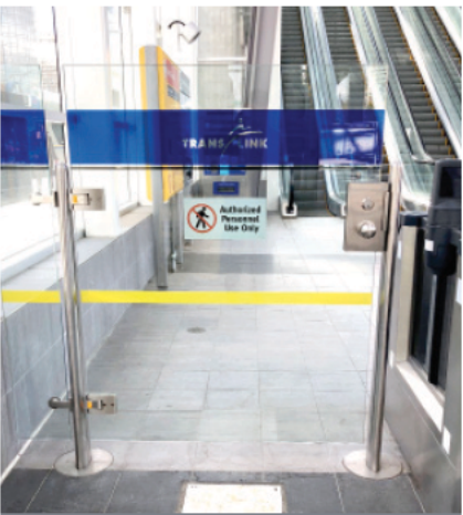
Fig 7.10 Example of an Equipment Gate
