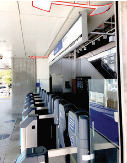
Fig 7.5 Example of Bi-Directional RFID Assemblies - RFID antennas are seen installed above the nearest and farthest faregate (outlined in red).
