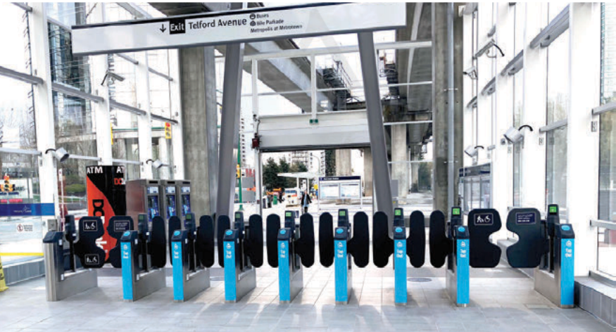
Fig 7.20 Example of Faregate Array Type 1 - Standard Bi-Directional Metrotown Station, Expo Line
