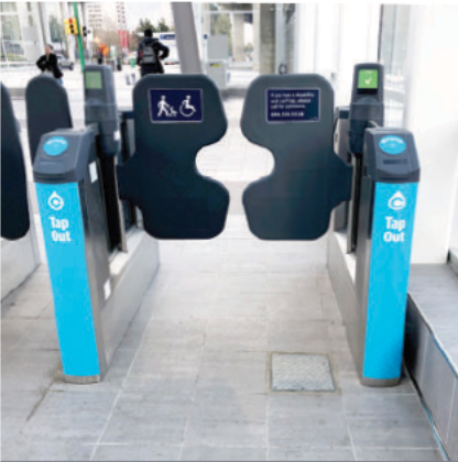
Fig 7.2 Example of an Accessible Faregate
