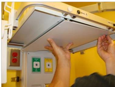
2. Remove the four screws and washers from the plate on the bottom shelf.
