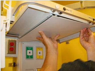
3. Remove the four screws and washers from plate on bottom of shelf.
