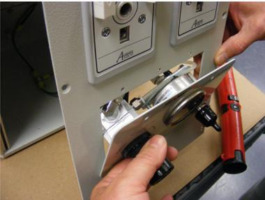
5. Replace the regulator and attach it to the Service Head back panel.
