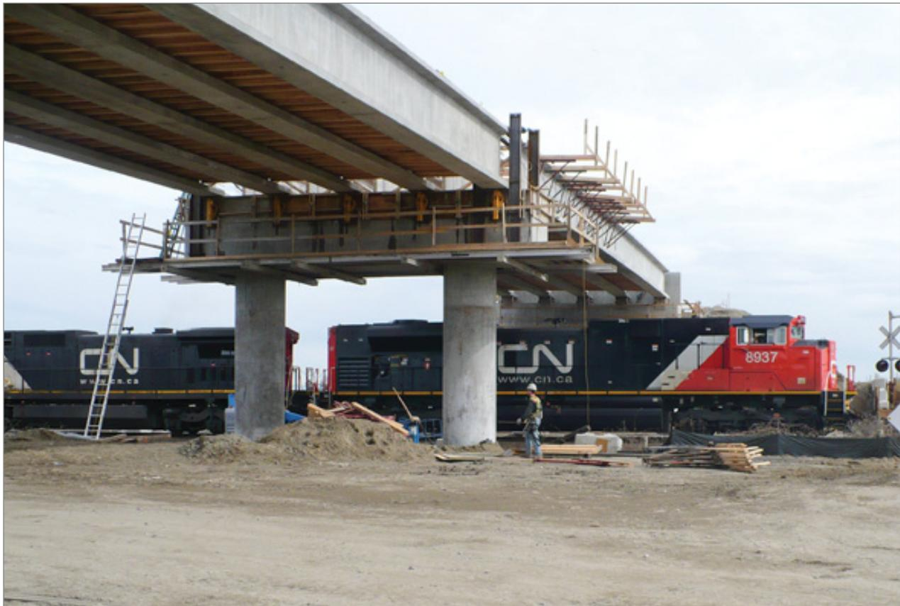
Construction of a new overpass to replace the existing at-grade rail crossing at 36th Avenue in Delta. The new overpass will allow continued access to farmland and local traffic flow.
